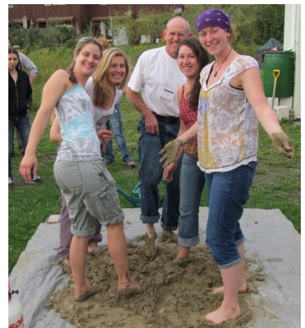
Students mixing sand, clay, and straw to make cob
